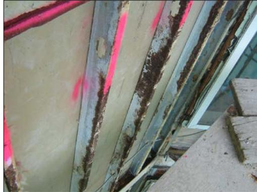
**FIGURE 3 - Extensive steel stud damage**
