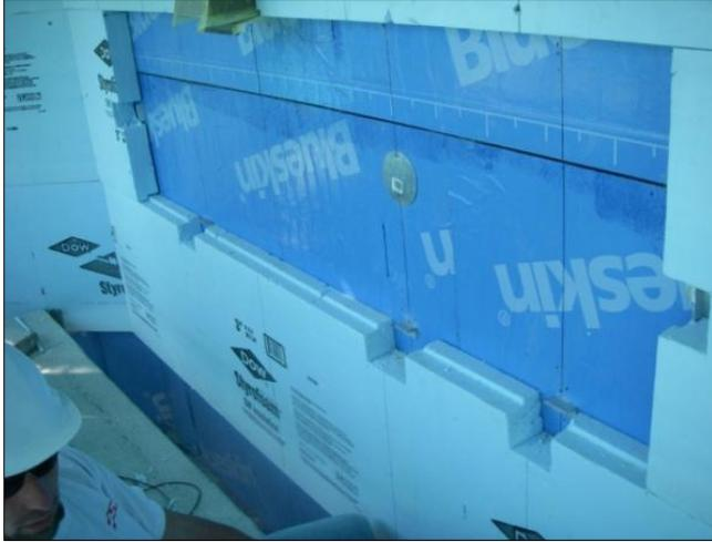
**FIGURE 14 - Measurement Panel Location Prepared for Board Installation**
