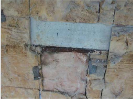
**FIGURE 4 – Semi rigid insulation with slab edge**
