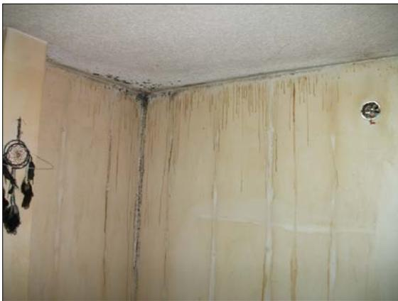
**FIGURE 6 - Interior Moisture Damage Related to Condensation and Leakage**
