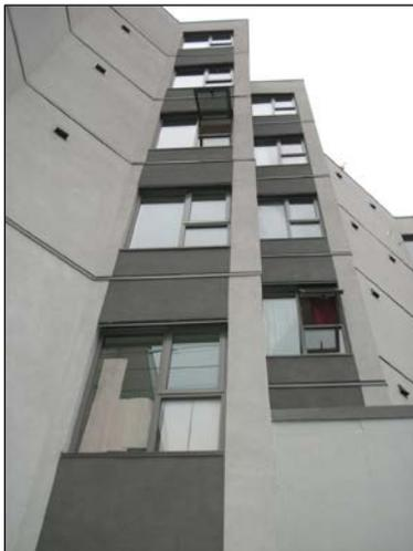
**FIGURE 9 - Completed Continuously Insulated Rain Screen Stucco System**
